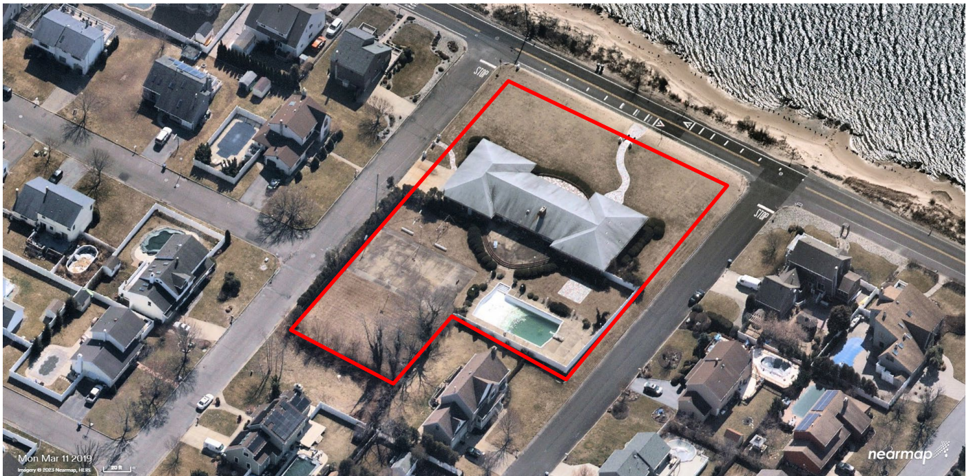
VIEW FROM NORTH
