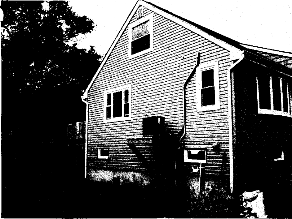
Flood Vents and side view (9/1/13)
