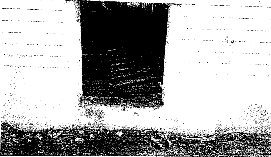
CRAWL SPACE ACCESS 105 MILFORD ROAD NEPTUNE, NJ 07753 DECEMBER 7, 2013
